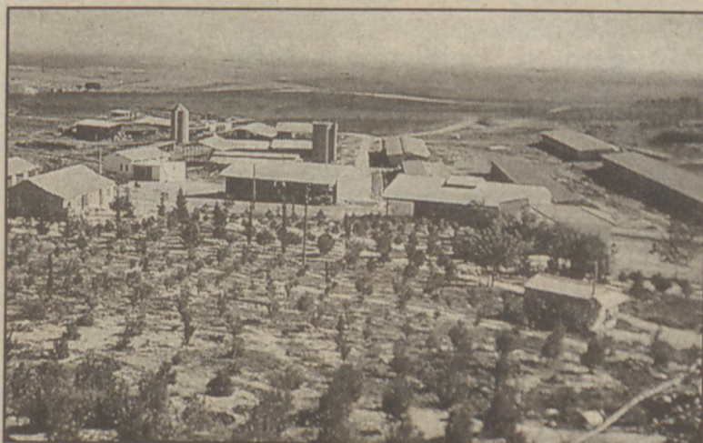
Kibbutz Shoval, partially funded by Delaware community, 1953.
