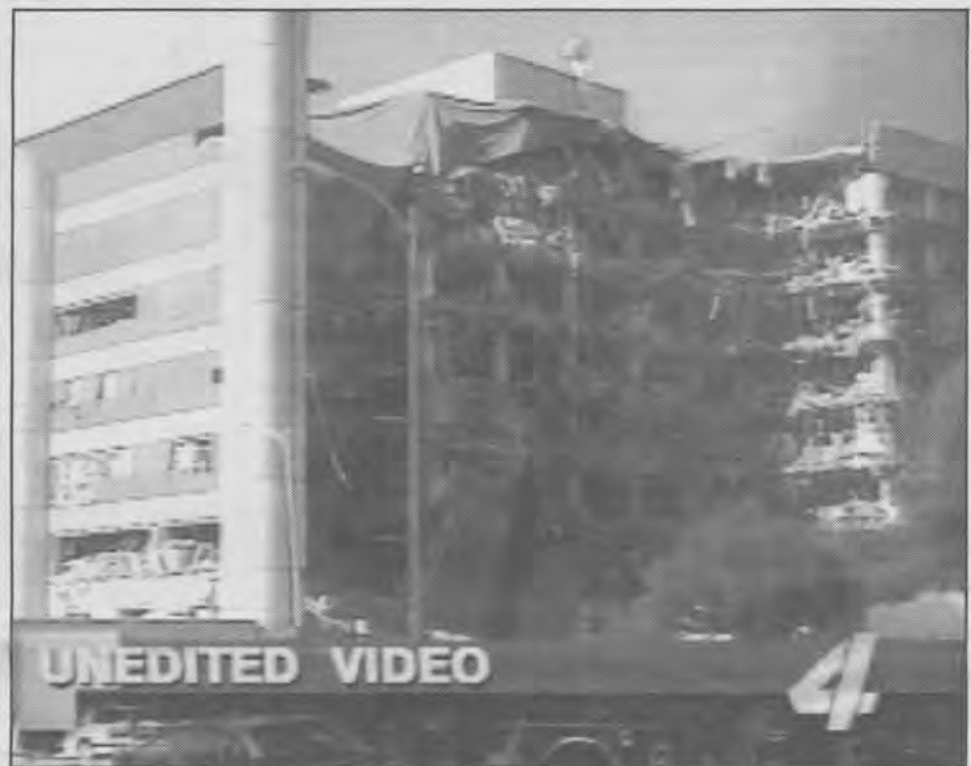
RNS PHOTO - Television coverage showed the devastation to the Oklahoma City federal office building.
