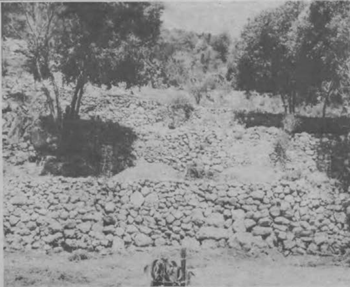
Terrace retainer walls developed by the Jewish National Fund at the experimental farm in Sataf (above) are helping a team of farmers examine the agricultural technology used during the time of King David, which enabled Jerusalem to prosper with its poor soil and limited rainfall. Hillsides are terraced with retainer walls made of stone. Run-off rainwater, which is not absorbed by the hard soil, travels down the hills and is captured in these terraces. The water then trickles down through the stones to each level, where it is absorbed by softened soil or channeled through hand-carved irrigation trenches directly to individual rows of vegetables. The staff at the Sataf farm now grows a large enough crop to feed itself and sell its surplus to the local Jerusalem markets.
