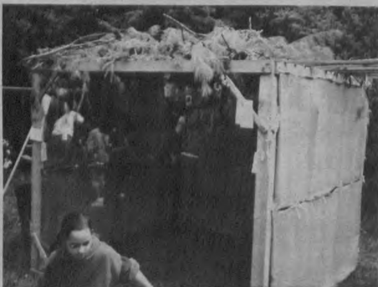
The Cowan-Lewittes family uses burlap for the sides of its sukkah . The frame is made from lumber that may be used from year to year.
