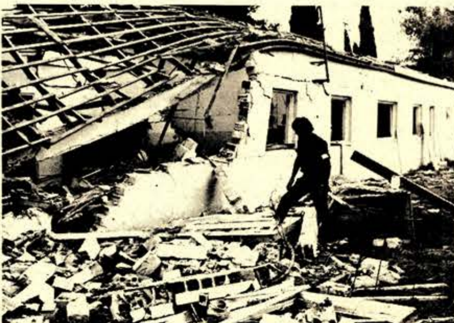
A Syrian "FROG" missile demolished this kindergarten building at Kibbutz Gvat.
