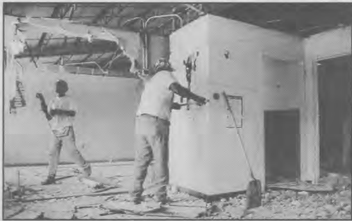
Construction workers at the Kutz Home. Photo: JDS
