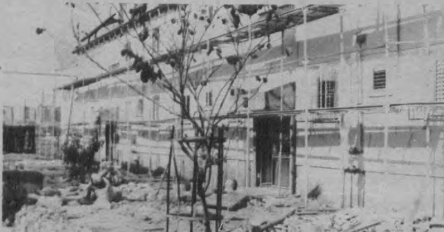
Jesse Cohen — Apartment building rehabilitation in progress
