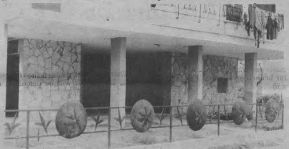
Improvement work in progress being done by residents
