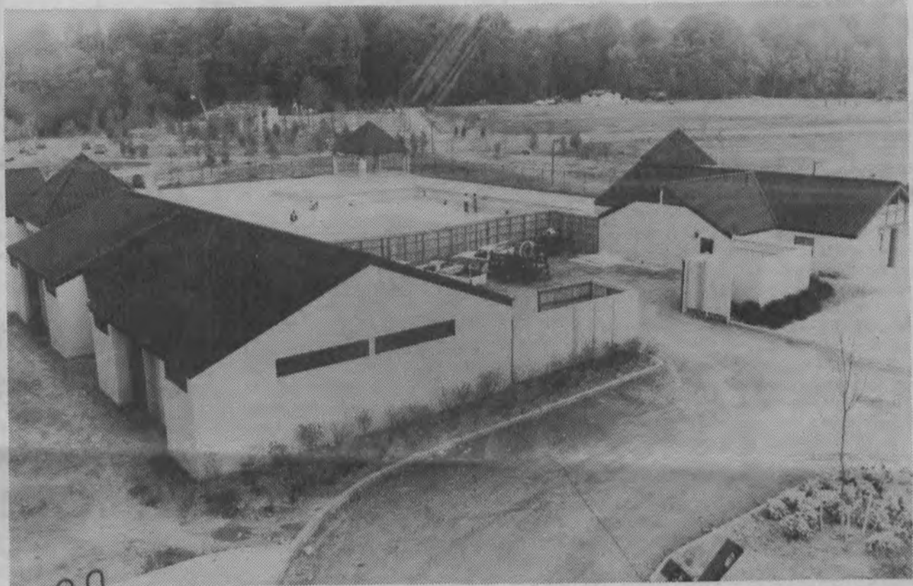
The new Family Campus buildings are nearing completion. The buildings shown will house the maintenance facilities and camp offices. The pool is in the background. The woods on the property will be used by the summer campers for a variety of activities, including hiking and nature study. (Photo credit: Brad Glazier)
